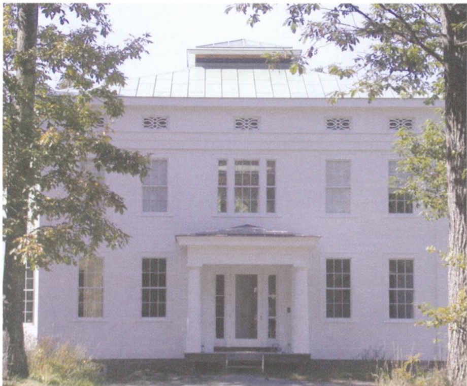
A Greek Revival Revival villa, with flush siding and fluted Tuscan portico columns, has arisen where a 1950s cabin once stood. Photo: Kate Johns
