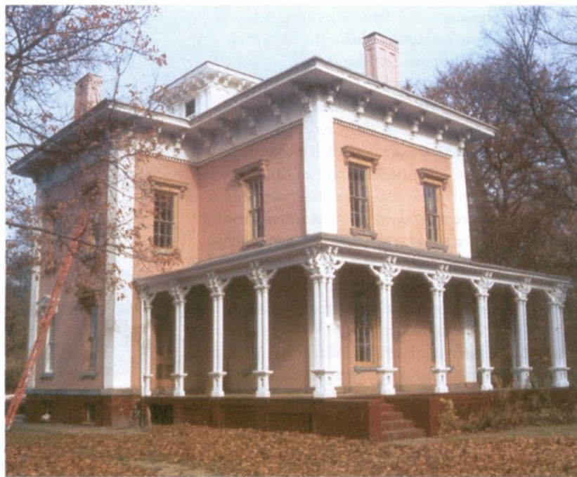
In restoring this brick 1840s Italianate, Johns discovered that its window sills were granite and the window trim carved mahogany. Photo: Christopher Billingham
