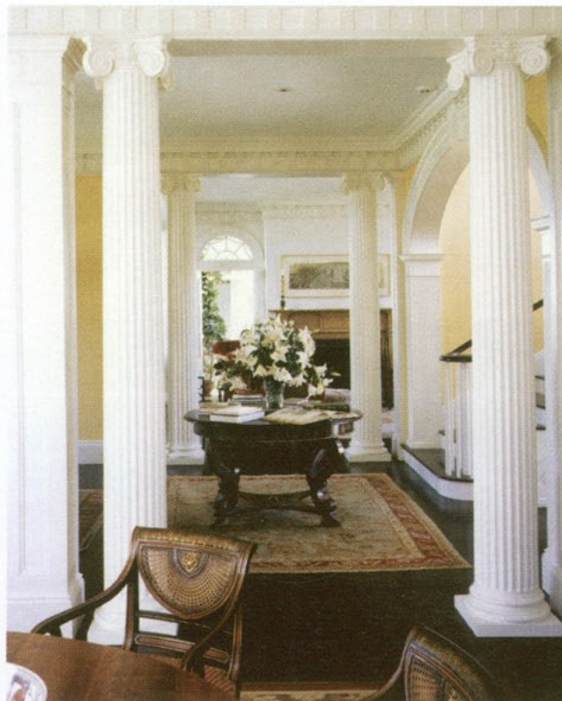
A mixture of stock columns and custom moldings ornament the house's enfilade of rooms. Photo: John M. Hall
